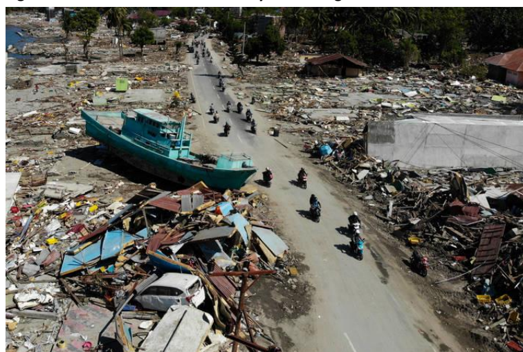
Figure 5.2: Stranded boat and destroyed buildings in Palu.
